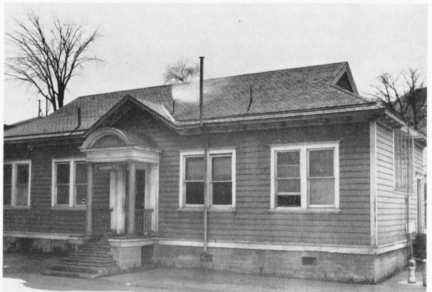
Built during World War 1 out of the best materials available, and kept in A-1 condition ever since, the East Plant Hospital, above, will soon be sold to the highest bidding employee or group of employees. The Company offered the building to employees with the hope that the materials available might help a few more people in building during the present shortage. The building is 56 by 26 feet, 1 1/2 stories high. (Story and building details on Page 1.)
